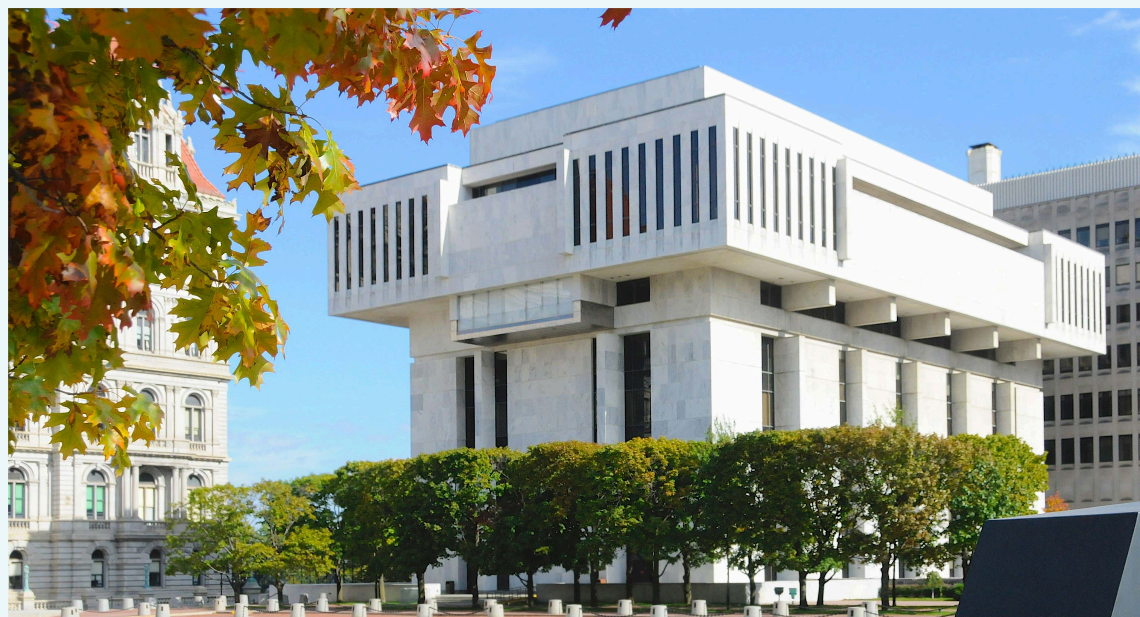
The Appellate Division, Third Department courthouse
